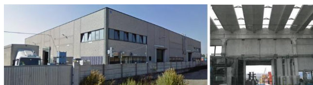
Figure 3. Type 3 (T3), buildings with long span planar roof: example of exterior and interior views.
