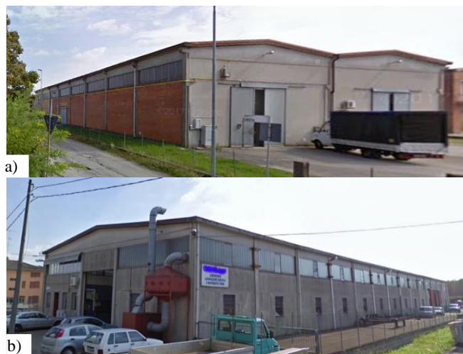
Figure 1. Type 1 (T1), Building with double slope precast beams simply-supported at the top of the columns and a) masonry cladding panels, b) horizontal precast cladding panels placed between the columns.
