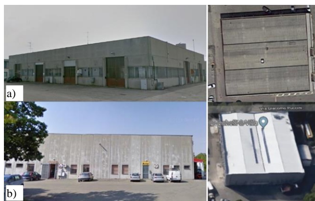
Figure 2. Type 2 (T2), buildings with double slope precast beams simply-supported at the top of the columns with external precast heavy cladding panels fixed externally to the columns a) horizontal panels or b) vertical panels.
