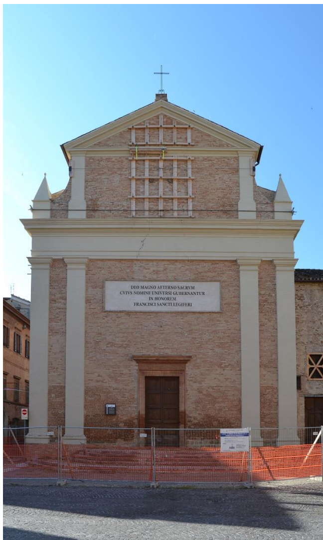
Figure 3. The façade of San Francesco in Tolentino (MC).
