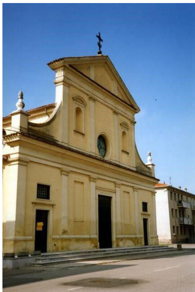
Figure 4. The façade of San Giovanni Battista in San Giovanni del Dosso (MN).
