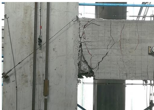
Figure 14. Tests on exterior joint: dissipative region.
