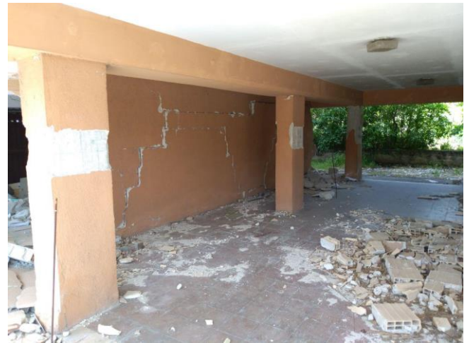
Figure 5. Example of a typical RC building with no partitions at the ground floor damaged by the L'Aquila earthquake (2009).
