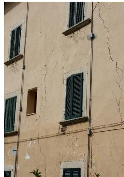
Figure 1. Cracking in historic building after earthquake: Pescara del Tronto, Italy.
