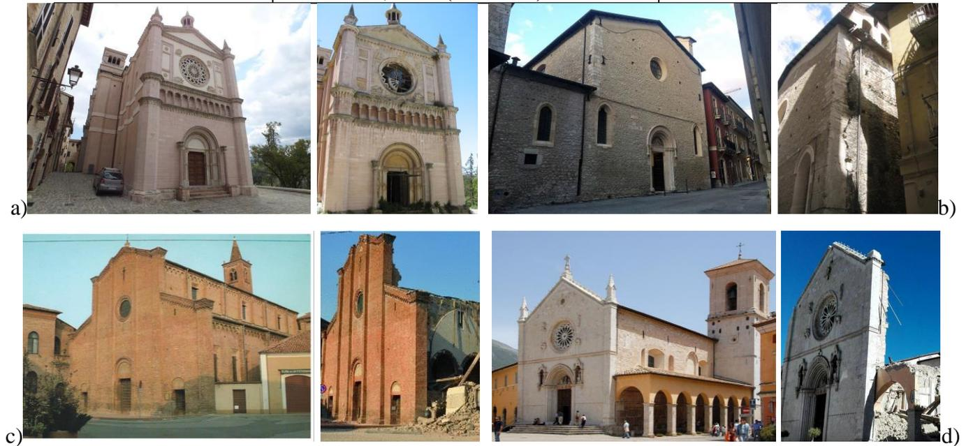
Figure 1. a) San Filippo Neri (Nocera Umbra): façade before and after the 1997 earthquakes; b) San Giuseppe dei Minimi (L'Aquila): façade before and after the 2009 earthquakes; c) San Francesco (Mirandola): façade before and after the 2012 earthquakes (courtesy of Andrea Penna); d) San Benedetto (Norcia): façade before and after the 2016 earthquakes.
