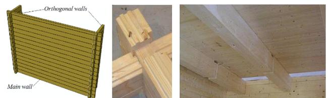
Figure 3. Example of Blockhaus system components: typical shear wall, with corner joint and inter-storey floor.
