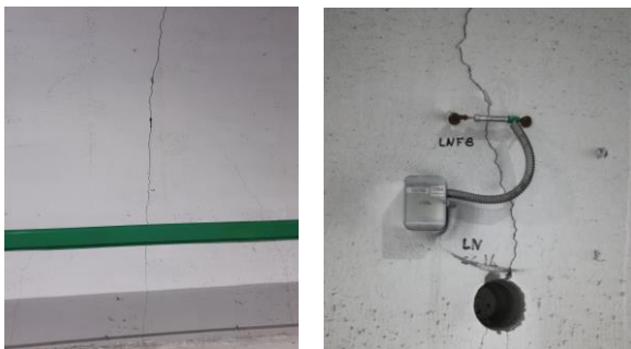
Figure 11. Monitored vertical cracks
