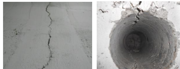
Figure 13. a) Longitudinal crack, b) checked by coring
