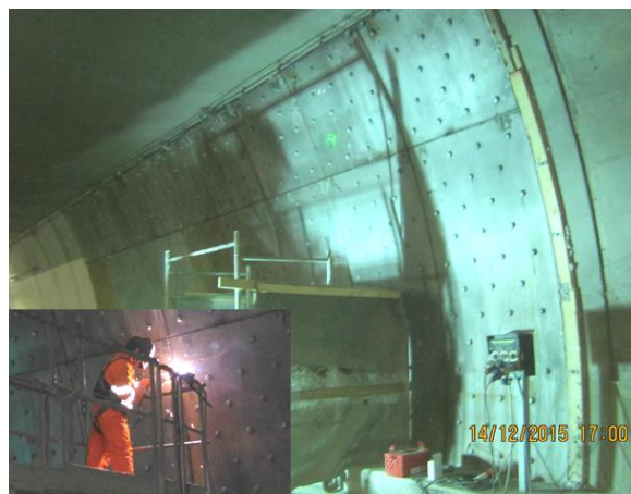
Figure 17. Reinforcement of sidewall by steel plates
