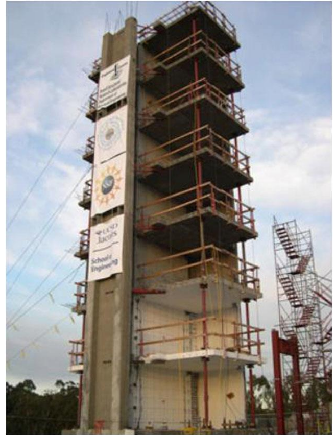
Figure 1. Test structure (Moaveni et al. 2010).
