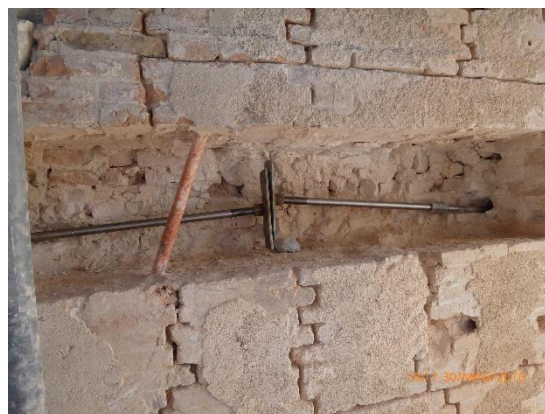
Figure 4: Steel retaining ties to prevent the main facade from overturning.
