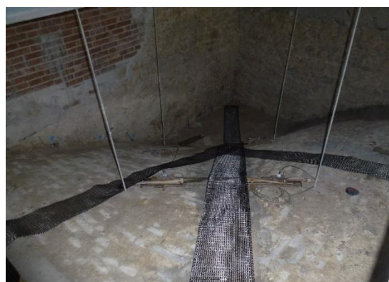
Figure 5: masonry vault strengthened at their extrados by carbon FRP strips.
