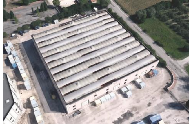
Figure 1. View of the industrial building of the Civil Protection Centre at Foligno, Italy.
