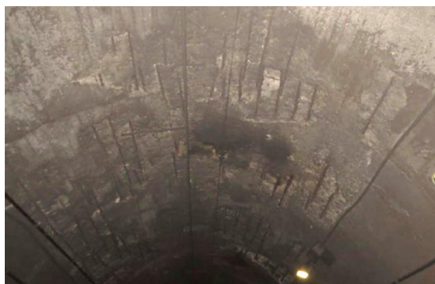
Figure 1. Example of degraded concrete tunnels (repertoire image).
