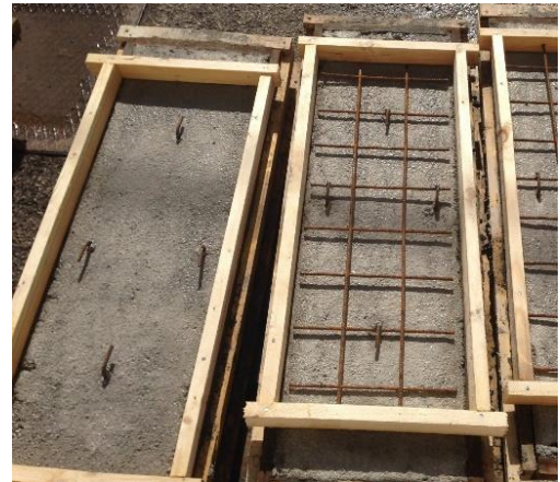
Figure 4. Installation of the electro-welded net and shear connectors.
