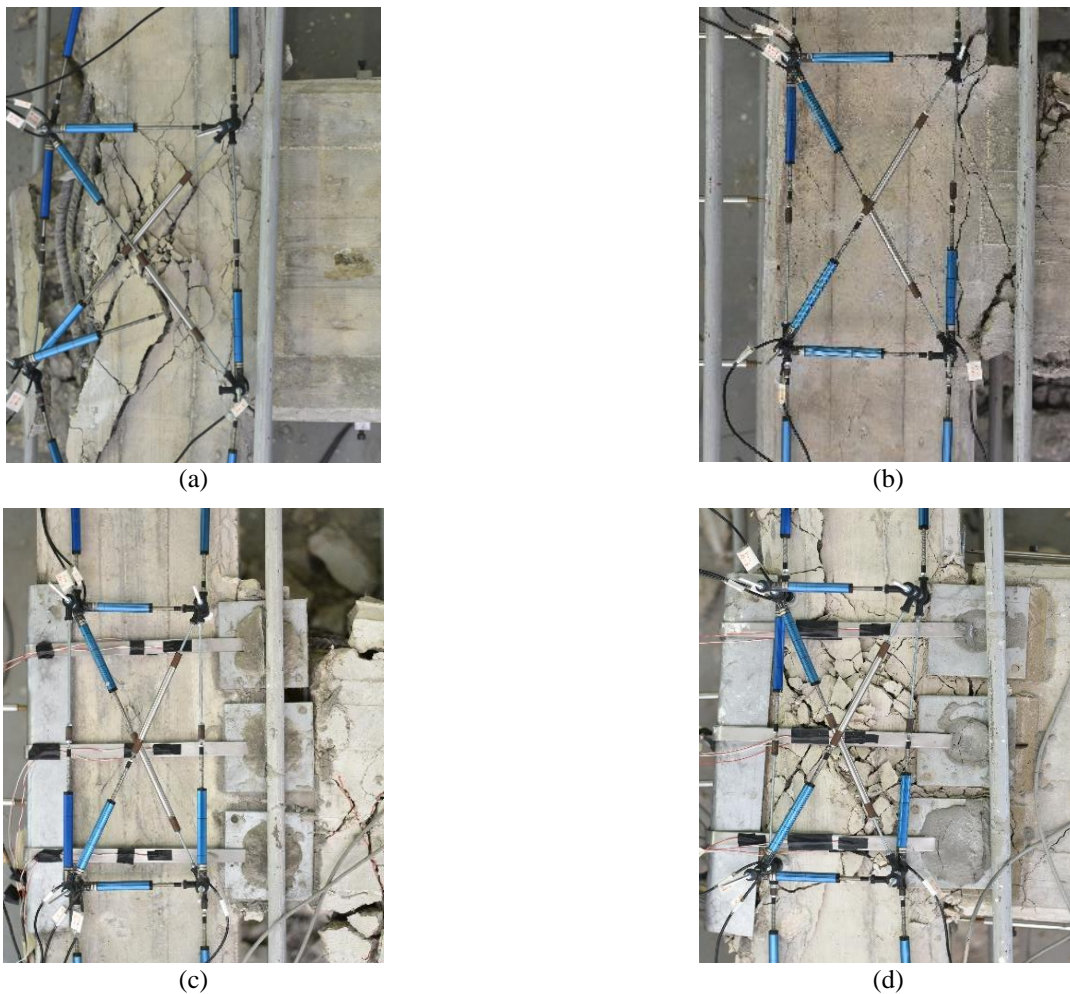
Figure 10. Observed damage at the end of test for tests 1NS (a), 1S (b), CAM1 (c), CAM2 (d).
