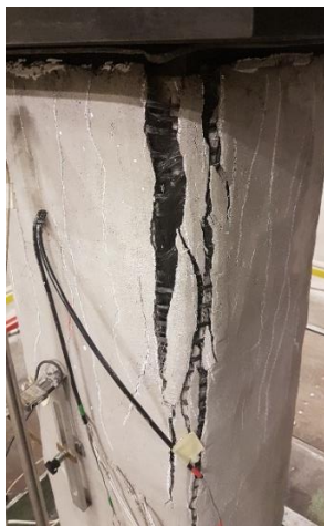
Figure 7. Cracks pattern development at the rounded edge with r = 20 mm (S33-2 specimen).
