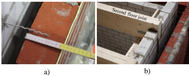
Figure 6. Connection details: a) inner-to-outer leaf with steel ties; b) timber beams-to-transverse walls with L-shape steel anchors.
