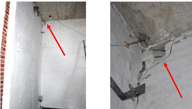
Figure 20. Bare building at ultimate conditions: first storey South-East corner.
