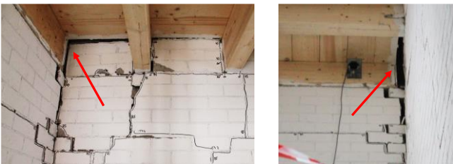
Figure 19. Bare building at ultimate conditions: second storey North-West corner.
