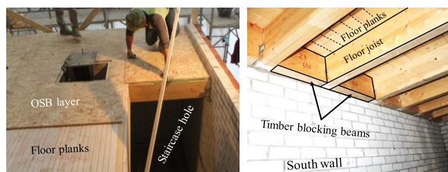
Figure 10. Stiffened timber diaphragm construction details.
