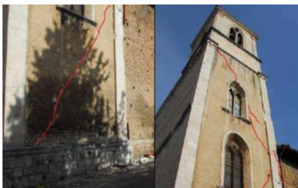
Figure 6- The two mechanisms of overturning
