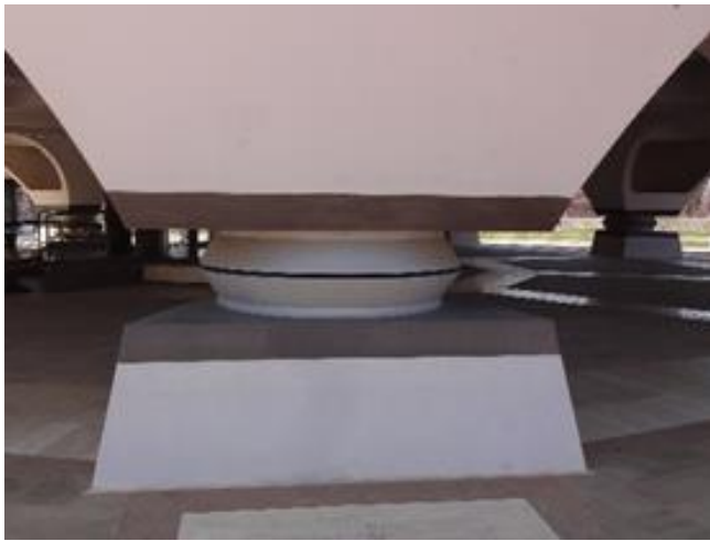
Figure 5. Support of an isolator after its completion
