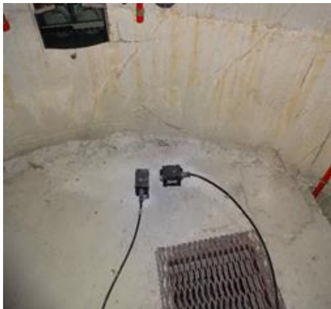
Figure 11. Accelerometers (A11 – A12) in internal core top.
