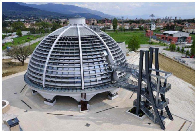
Figure 3. Operation room building
