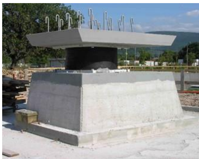
Figure 4. Support of an isolator during the construction
