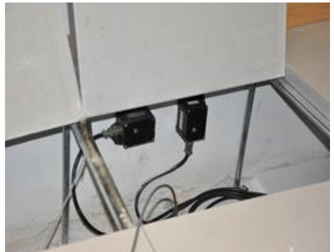
Figure 10. Accelerometers (A04 – A07) below the floating floor
