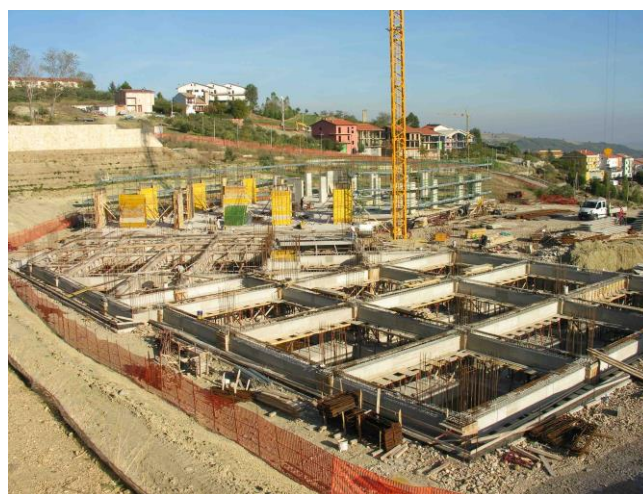
Figure 2. The isolated deck of the two-block school building at San Giuliano di Puglia, Italy, during the construction.
