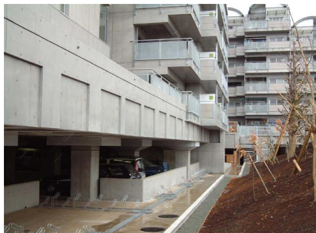
Figure 1. Lateral view of a complex of twenty one 6- to 14-storey buildings, all erected on an unique artificial ground at Sagamihara, Tokyo.
