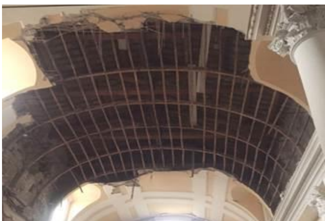
Figure 5. Examples of reed-mat vaults: a) Santa Chiara (Camerino).
