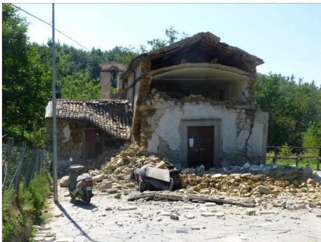
Figure 4. Example of poor quality masonry causing wall disintegration: San Lorenzo Martire (Cossito, Amatrice)
