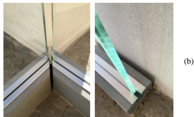
Figure 5. Foundation system. (a) Cross-sectional drawing and (b) detail views (drawing and photos by A. Danelutti).
