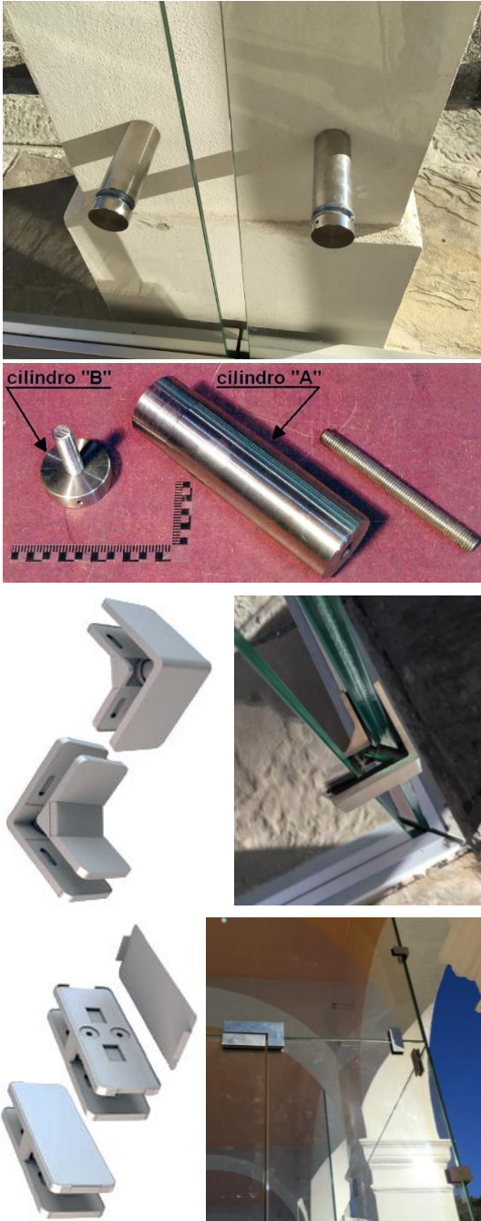
Figure 6. Elevation restraints. (a) Glass-to-building connectors and (b) glass-to-glass friction clamps for corners or (c) overlapping panels (photos by A. Danelutti and F. Trevisan).
