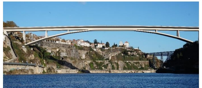
Figure 3. Deck stiffened arch system applications : Infant Dom Henrique Bridge by A. Adão da Fonseca, 2002
