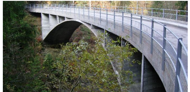
Figure 2. Deck stiffened arch system applications Schwandbach Bridge by Robert Maillart, 1933
