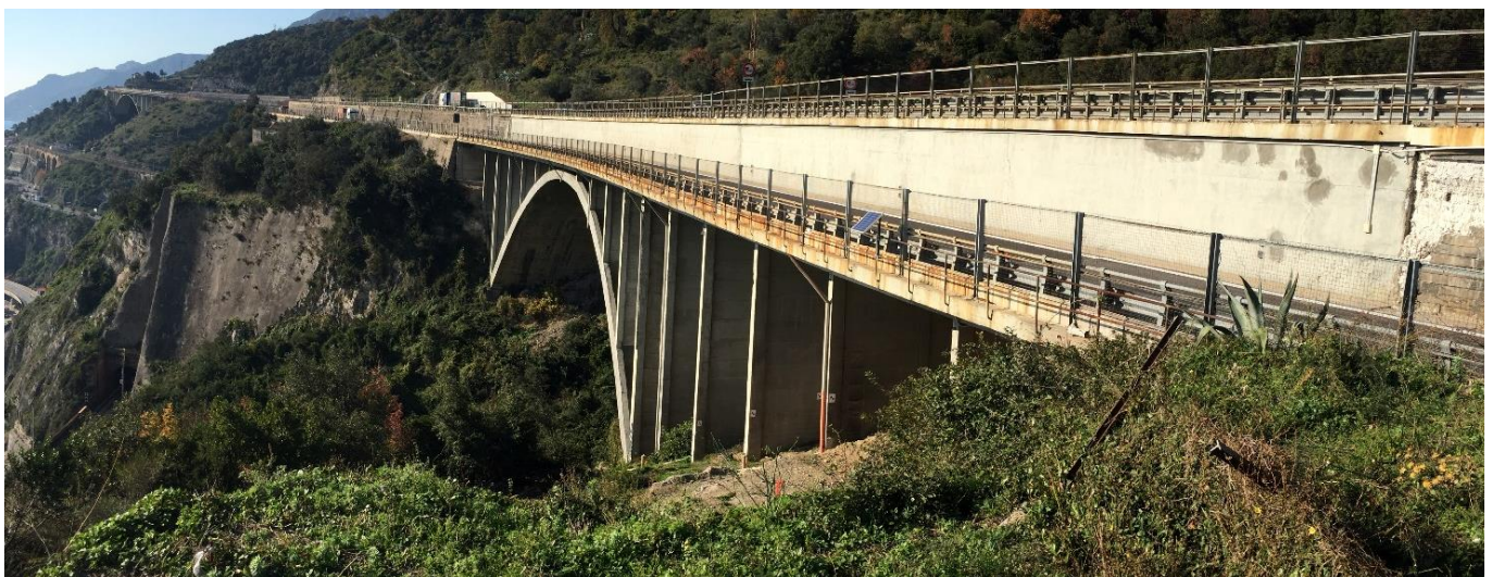
Figure 5. Olivieri Bridge general layout: Maillart arch bridge with staggered carriageways (“Z-shaped” deck)
