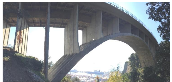
Figure 7. Olivieri Bridge details: cross wall layout between the upper deck and the lower arch
