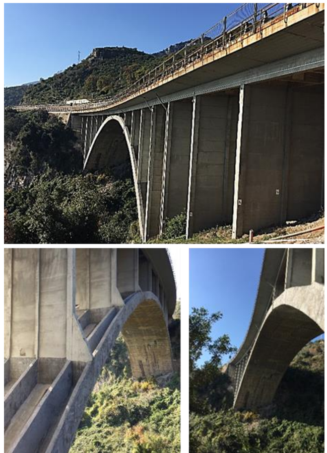
Figure 2. Olivieri Bridge layout and detail of ribbed vault
