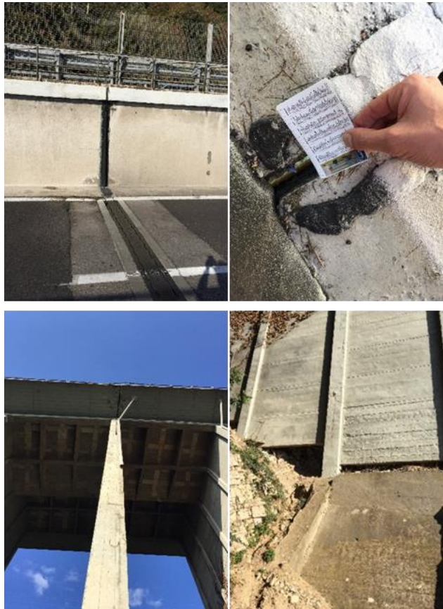
Figure 3. Olivieri Bridge: joint section (above); cross walls detail at the joint section and attach to foundation (below)
