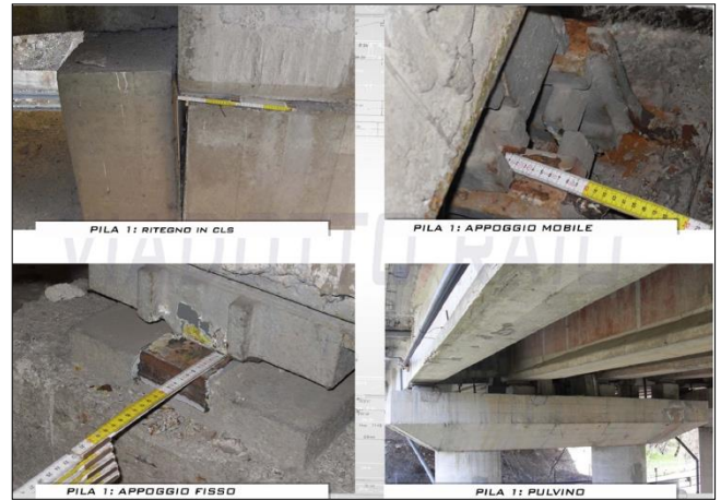
Figure 6. Damage to abutments bearing devices in Raio e Aterno viaducts after April 6, 2009 L'Aquila earthquake (SDP 2019b).
