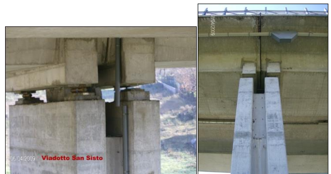
Figure 7. Damage to girder-deck viaducts after April 6, 2009 L'Aquila earthquake (SDP 2019b).
