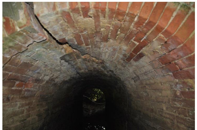
Figure 10 Longitudinal crack on the vault of the bridge
