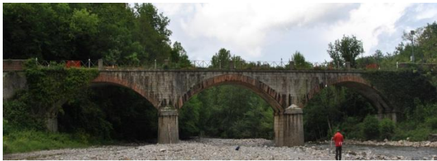
Figure 5 Masonry vault bridge
