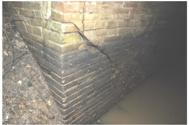
Figure 9 Diagonal crack on an abutment of the bridge
