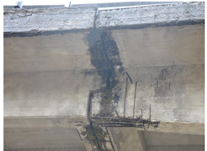
Figure 2 Degradation, spalling and corrosion in correspondence of a Gerber saddle
