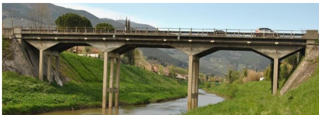
Figure 6 Gerber beams bridge
