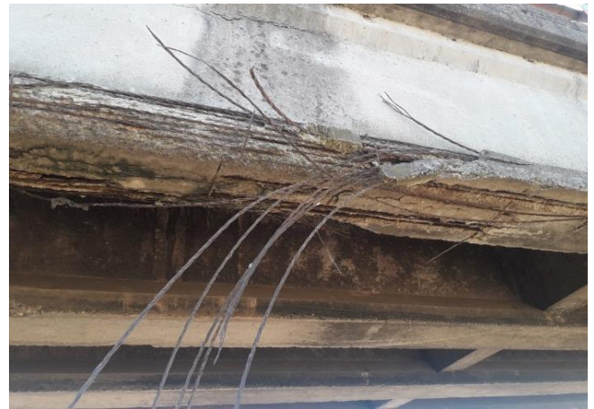
Figure 1 Breaking and leakage of pre-stressing reinforcement bars
