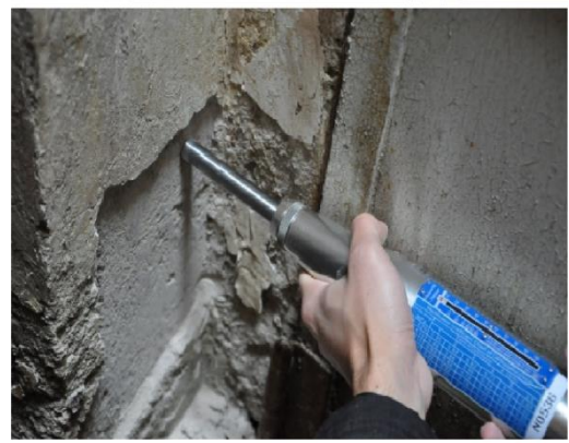
Figure 6. Constructional element identification using concrete hammer test
