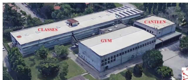
Figure 3. Building overall view
