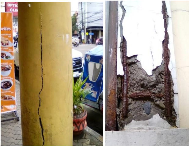
Figure 5. Damaged columns: deep vertical cracks (left); concrete cover crushing (right).
