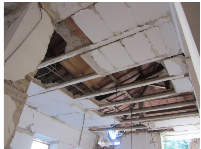
Figure 3. Damages in wing “B” after the seismic sequence: out of plane collapse of a corner (top), partial collapse of the attic floors (bottom).
