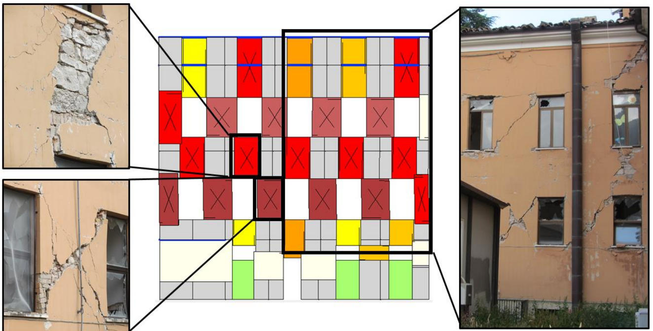
Figure 10. Comparison between the damage obtained from the numerical simulation and the one observed on the building at the end of the seismic sequence, wall 4 of wing "B".
